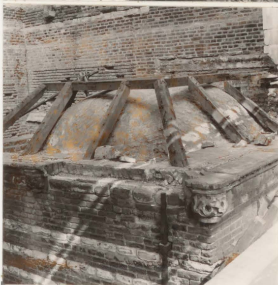
NEG.NO. 112. OCT. 1966. PILASTER IN WESTVLAK STEUNBEER 95.
